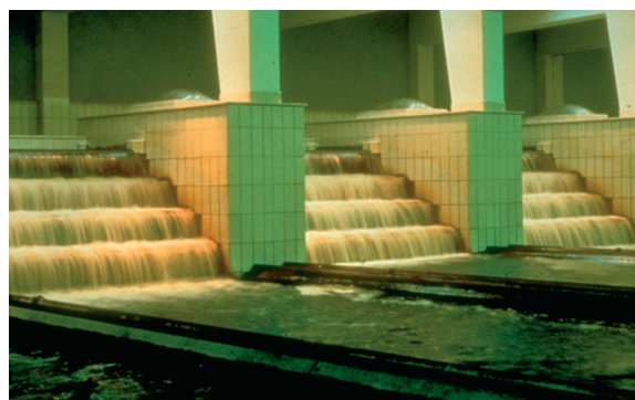
Figure 4 - Aeration and submerged granular media filtration at the Noord-Bergum pumping station (Friesland)
