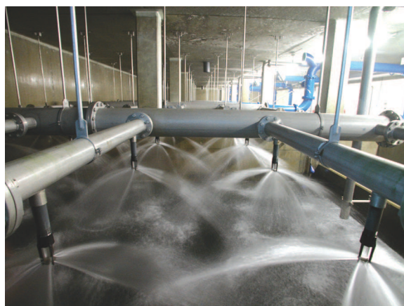
Figure 9 - Aeration over a dry filter in Zwijndrecht (Zuid-Holland)
